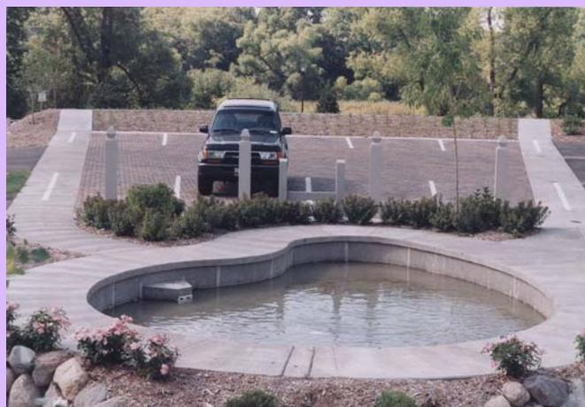
Pervious pavement like the surfaces at the Minnesota Landscape Arboretum's Rain Water Runoff Model illustrate a key element of Low Impact Development: surfaces specially designed and engineered to prevent, rather than capture or direct, stormwater runoff.
