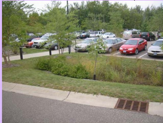
Vegetated swales at the HB Fuller Company Parking Lot in Vadnais Heights, MN, reduced stormwater runoff by 73%, phosphorus by 70%, and sediment by 94%.
