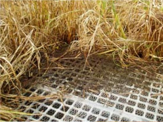
The pictures show an overflow being covered by vegetation. This vegetation should be trimmed back and the overflow cleared.
