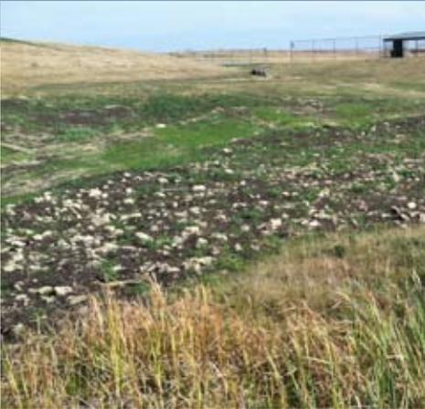
To the left is a picture of a raingarden project that will break up clay soils that have been compacted via the use of deep rooted prairie grasses. The large light colored chunks in the picture is clay that was mixed with compost (the dark brown soil) to allow for infiltration.
