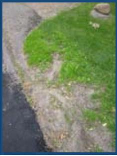
Erosion or gullies are when the soil is exposed and channels are created by flowing water. This exposed soil is now easily washed away and creates a dysfunctional BMP. This happens because water is flowing into the BMP faster than the design predicted, and is not holding up to large amounts of fast moving water. It can also indicate that water is entering the BMP in ways that were unintended by the design. This is a very significant indicator that your BMP needs maintenance.
