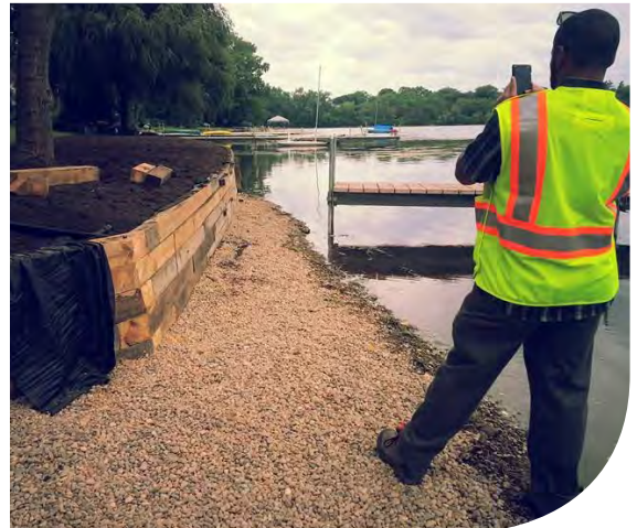
Figure 1.40 Staff inspecting a retaining wall
