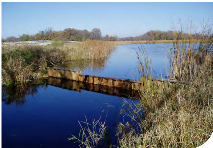
Figure 1.115 Painter Creek weir
