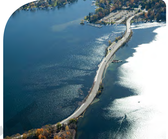
Figure 1.44 Bushaway Road shoreline project
