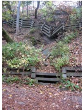
Failing wall.
